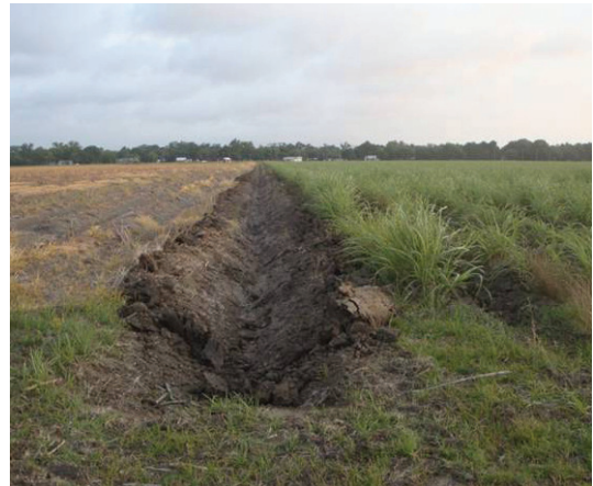
Mechanically cleaned drainage ditches (split ditches) increase erosion
